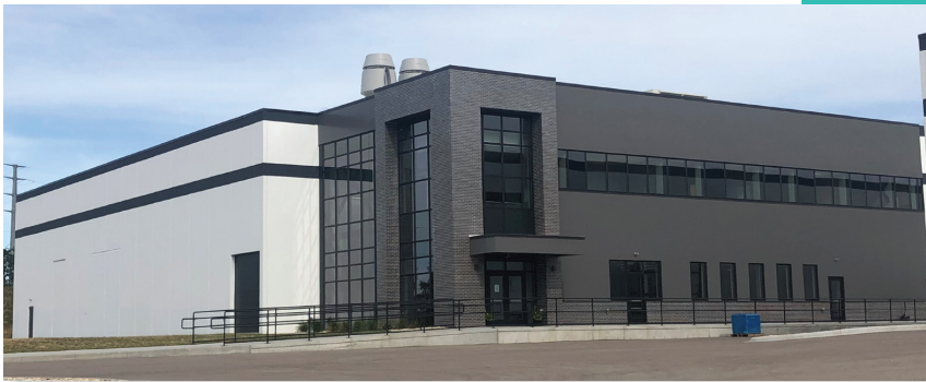
Dedicated 28,000 sq ft Cu-67 Accelerator Production facility
