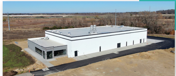
Dedicated 30,000 sq ft Ac-225 Production facility
